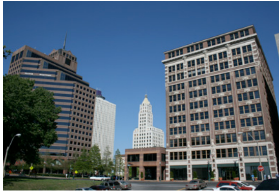
TOWERING CONTRACT: Commercial Alliance Management LLC was selected by Jackson, Miss.-based Parkway Properties Inc. to handle all new leases for its Downtown portfolio, which includes the Morgan Keegan Tower (far left) and Falls Building (far right). -- PHOTO BY ERIC SMITH
